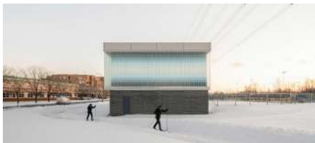
Water Intake of the Aqueduct Canal (2021) Photography by David Boyer
