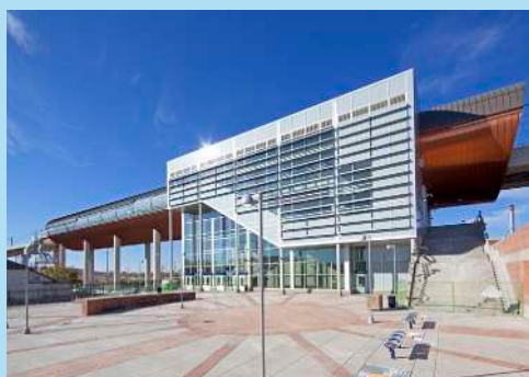
Sunalta LRT Station & Elevated Guideway
