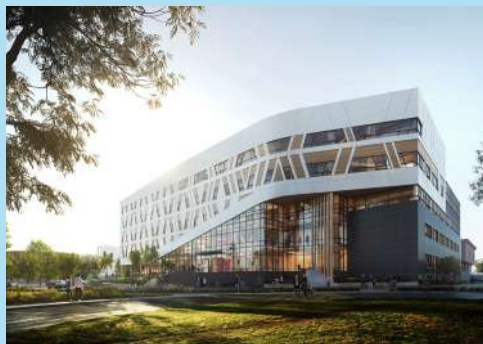
Centennial College A-Building Expansion
